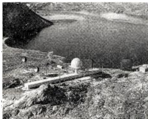
DEW LINE STATION on Baffin Island is part of the largest single defense system ever constructed—an operating radar system across the top of North America, having its own communications network.
